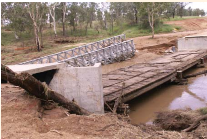
Recent construction in 2010 of Derarabungy bridge on the Beeron Road, destroyed.
