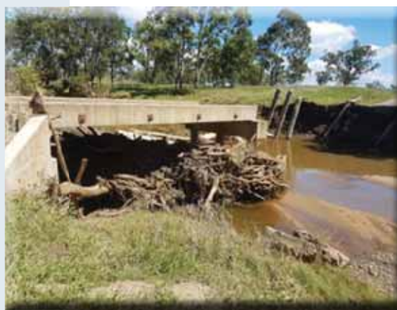
Percy Hindmarsh Bridge on Glencoe Road, Monto damaged as a result of Tropical Cyclone Debbie
