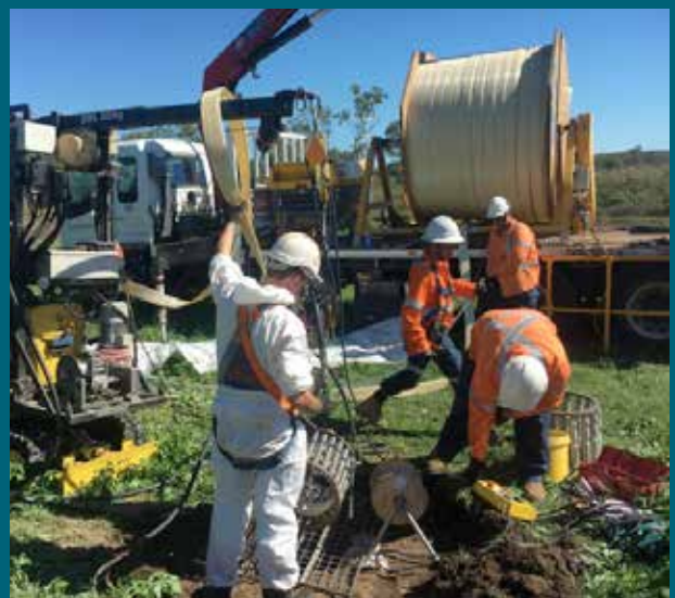
Commencement of the spiral wound sewer relining project at Monto
