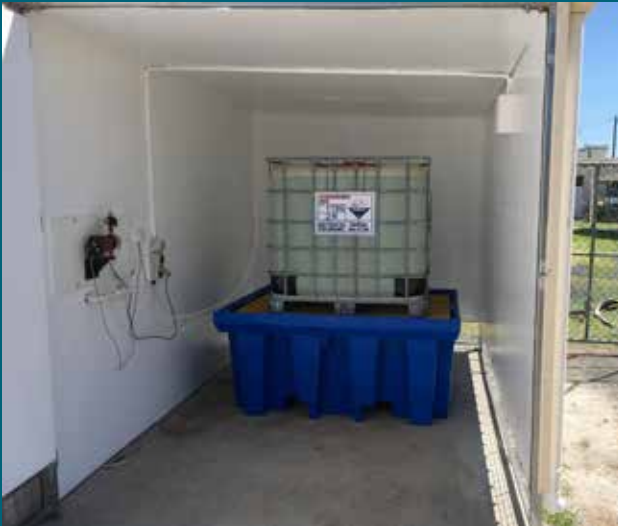
Top left: Monto pool acid dosing room
