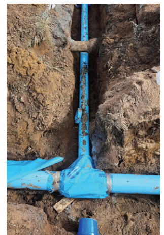
Above left to right: Mundubbera Water Treatment Plant effluent irrigator in action. Water mains being replaced.
