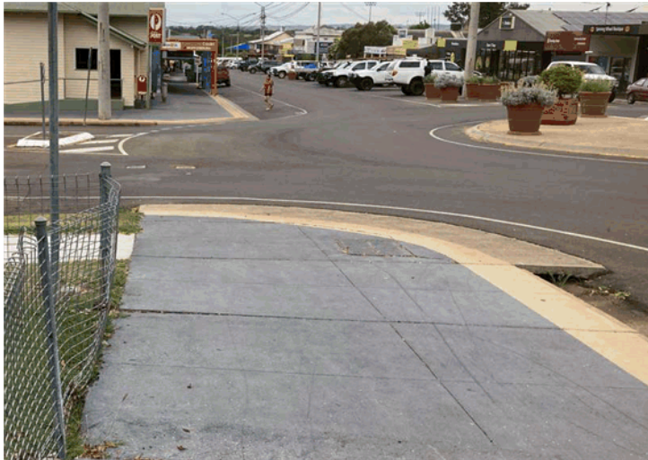
Ramps at Lyons St roundabout
