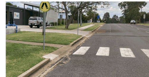
Fielding St - Missing path connections at school
