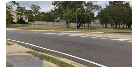
Bridge St / Dalgangal St intersection
