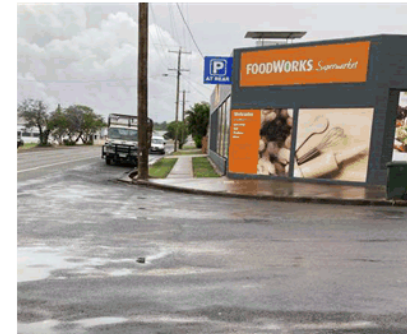
Missing kerb ramps, Lister St
