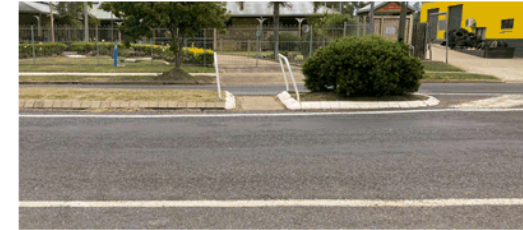
Capper St crossing point - shrub potentially obscures pedestrians
