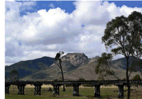
The PWP includes a connection to the start of the Bluff View walking track
