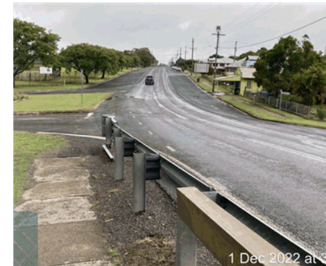
Connections to the rail overbridge path
