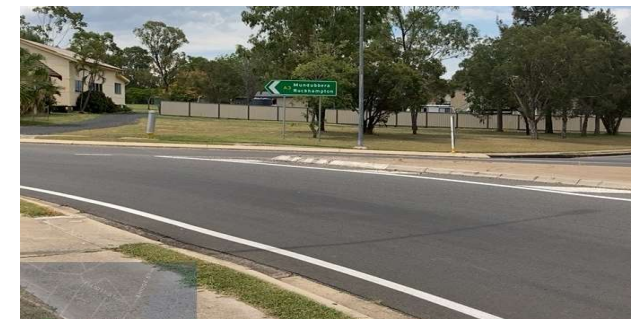
Bridge St / Dalgangal St intersection
