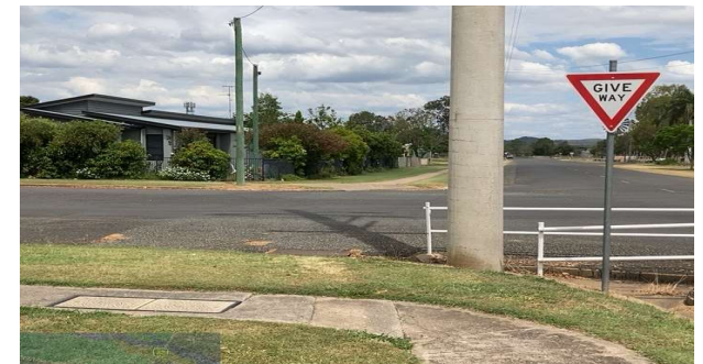
Example of poor path connections at an intersection
