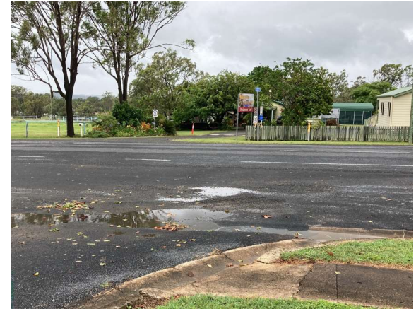
Showground and caravan park
