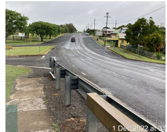
Connections to the rail overbridge path
