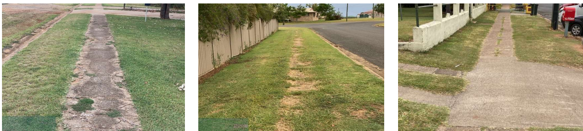
Examples of paths in poor to very poor condition, impacting on use by wheelchairs, prams etc
