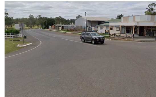
No kerb ramps – Burnett Hwy and Moreton St
