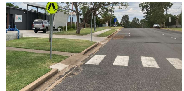
Fielding St - Missing path connections at school
