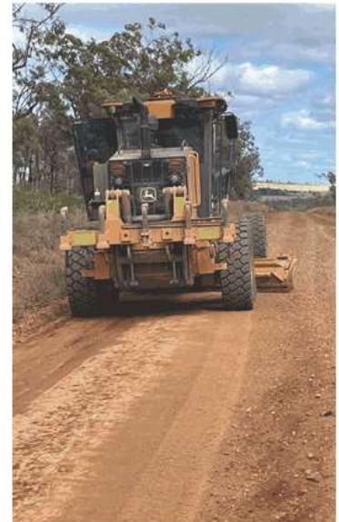
Above: Grading on Hawkwood Road.
