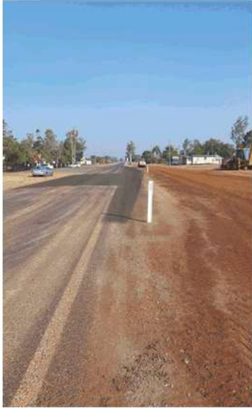
Above: Coalstoun Lakes Safe School road widening; finished project.
