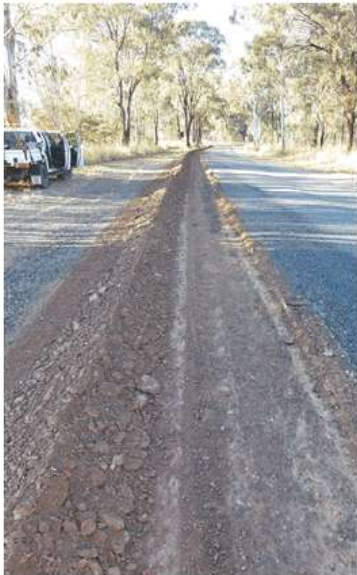
Above: Shoulder repairs on the Biggenden - Gooroolba Road; shoulders boxed out.
