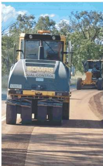
Above: Mount Perry Road stabilisation: Multi tyre roller in front of grader doing the final trim, steel flat drum roller.
