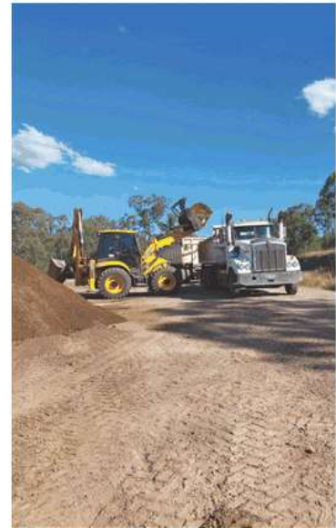
Above: Dulong Road shoulder repairs: Trucks being loaded with road base.
