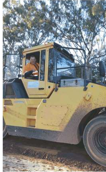
Above: Coalstoun Lakes Safe School road widening with multi tyre roller.
