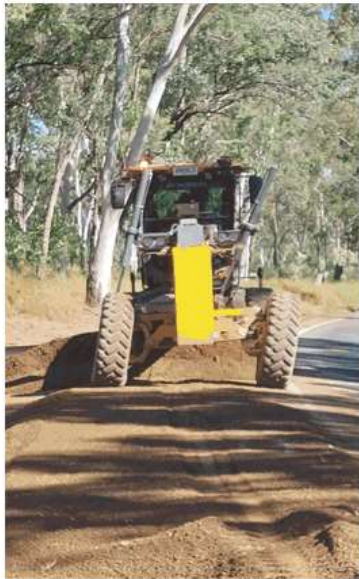
Above: Dulong Road shoulder repairs: Grader trimming road base.
