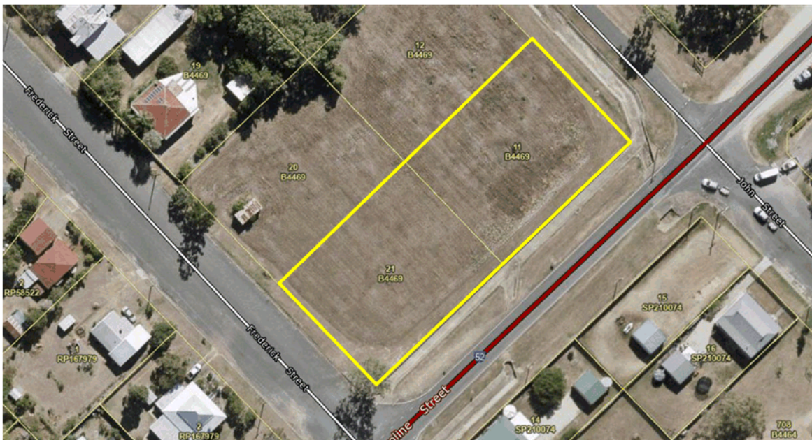
FIGURE 2-1: SUBJECT SITE AERIAL IMAGE (QLD GLOBE 2022)
