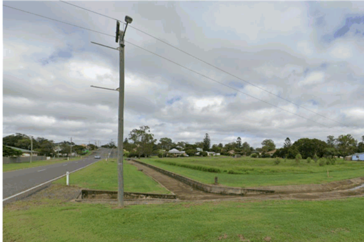
FIGURE 5-2 OVERHEAD ELECTRICAL – JOHN STREET
