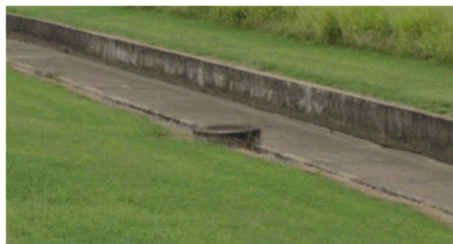
FIGURE 4-1 EXISTING SEWER MANHOLE WITHIN DRAIN
