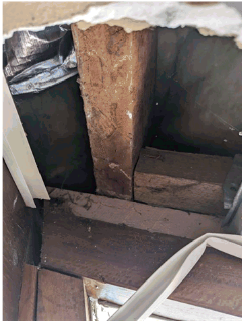
Photo 17 – Minor movement noted to raking timber member at top of front wall
