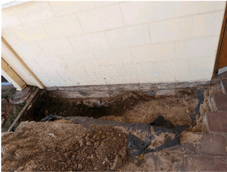
Photo 21 - Pavers and plastic removed left of front door. Previous grout injection repairs evident
