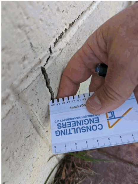
Photo 5 – Masonry crack with lateral movement
