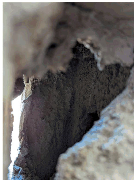
Photo 16 – Masonry crack at top of front wall. No corefill to block
