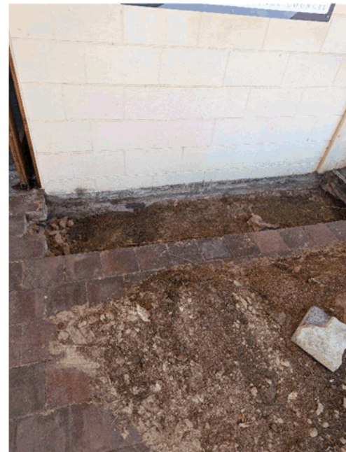
Photo 20 – Pavers and plastic removed right of front door. Previous grout injection repairs evident
