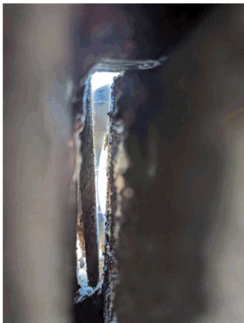
Photo 15 – Daylight through Masonry crack at top of front wall
