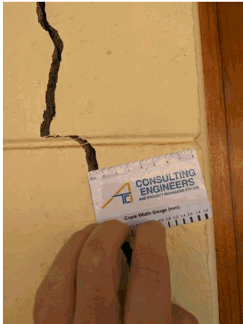
Photo 3 – Masonry crack near front door
