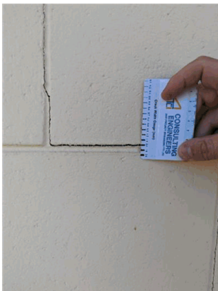
Photo 7 – Stepped Masonry crack
