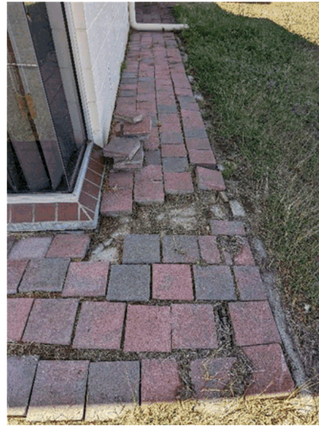
Photo 6 – Uneven pavers around building
