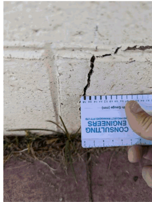
Photo 4 – Masonry crack near ground level
