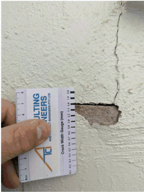
Photo 9 – Actual crack width disguised by render
