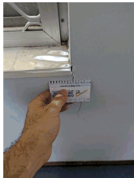
Photo 8 – Internal Crack in masonry and render
