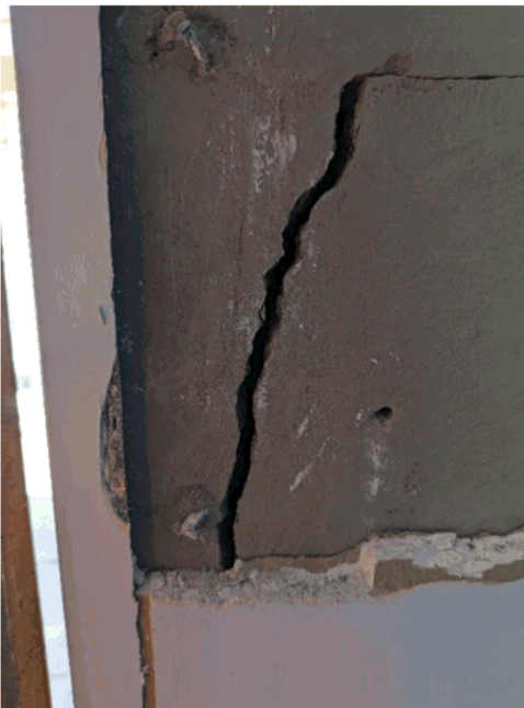
Photo 19 – Large masonry crack disappears behind plasterboard lining
