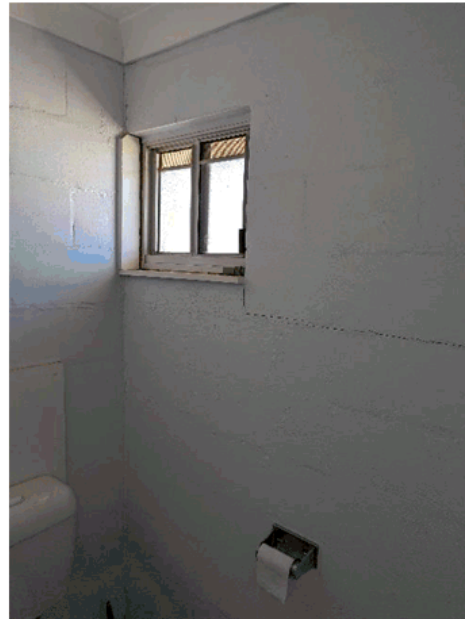
Photo 10 – Horizontal crack in bathroom wall
