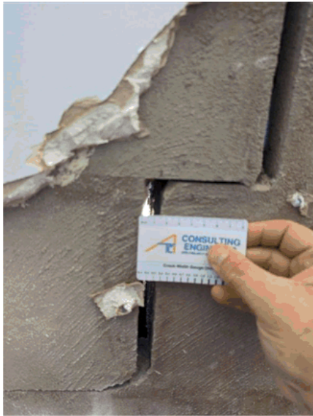
Photo 13 – Crack through masonry at top of front wall
