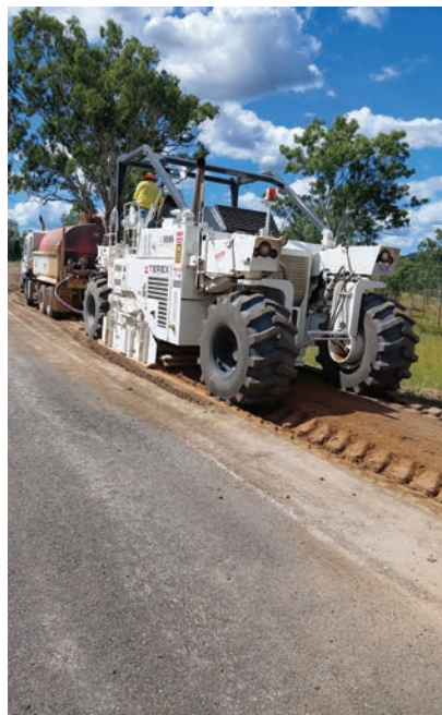
Above: Mount Perry Road stabilisation: Stabiliser and water truck in action.
