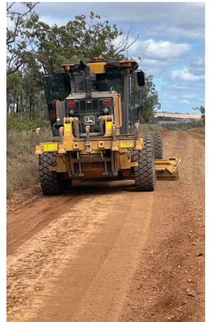
Above: Grading on Hawkwood Road.
