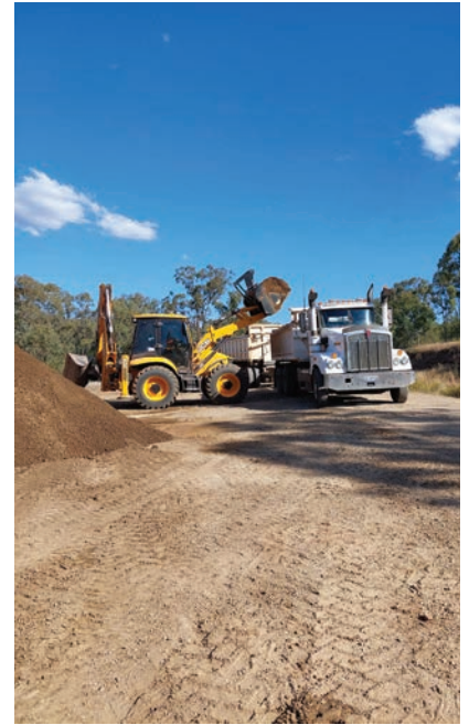
Above: Durong Road shoulder repairs: Trucks being loaded with road base.
