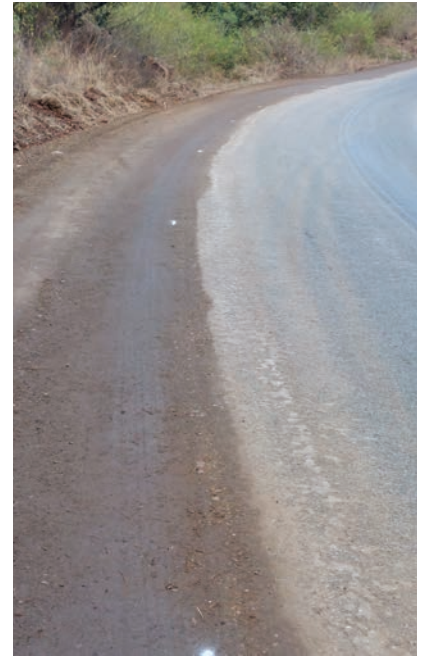
Above: Biggenden Mines Road shoulder repair: finished and marked out for bitumen seal.
