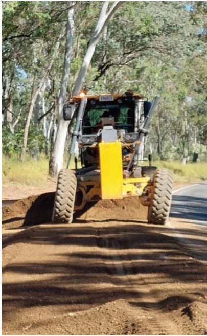
Above: Durong Road shoulder repairs: Grader trimming road base.
