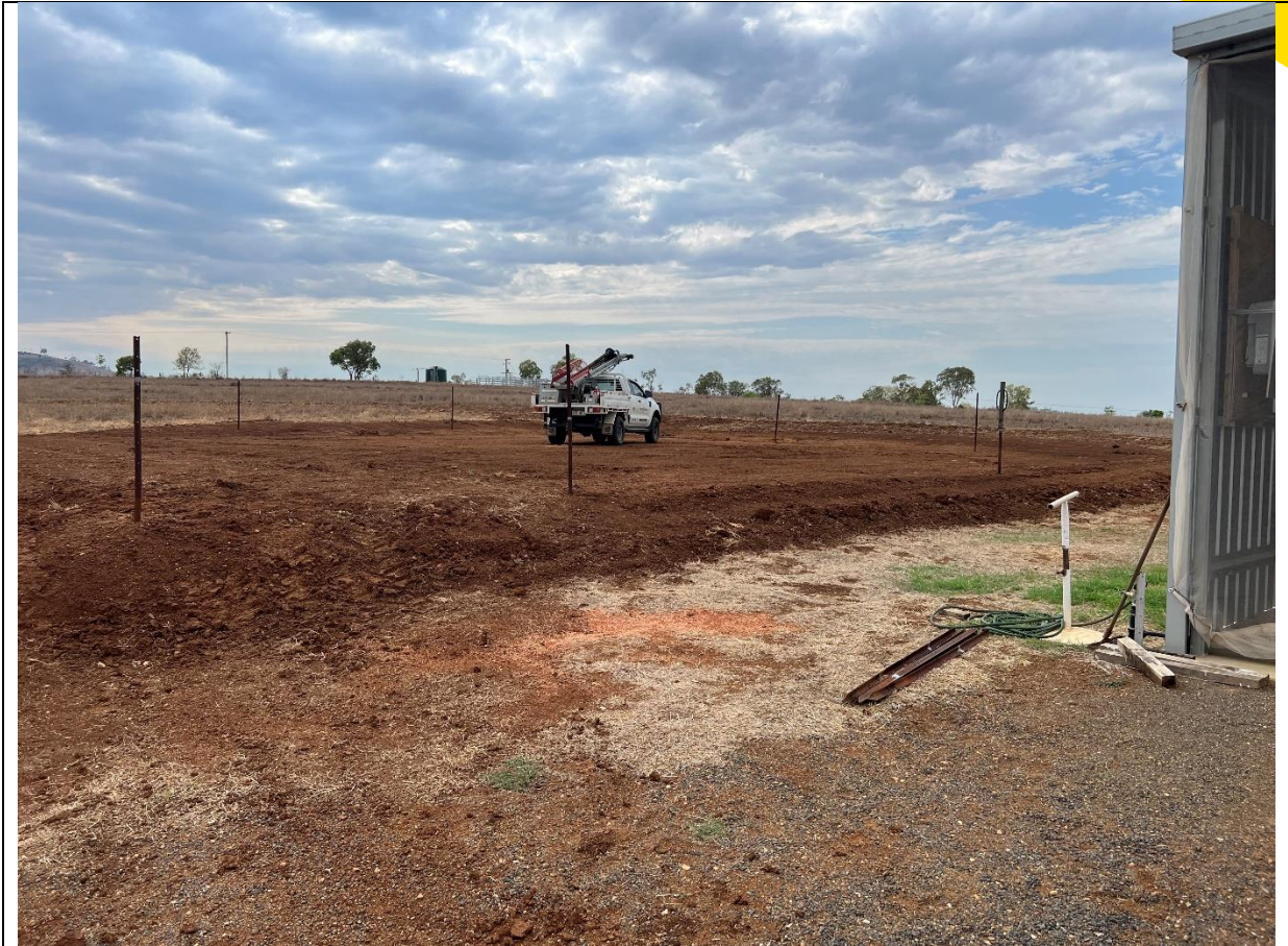
Image 1 – Proposed construction site
