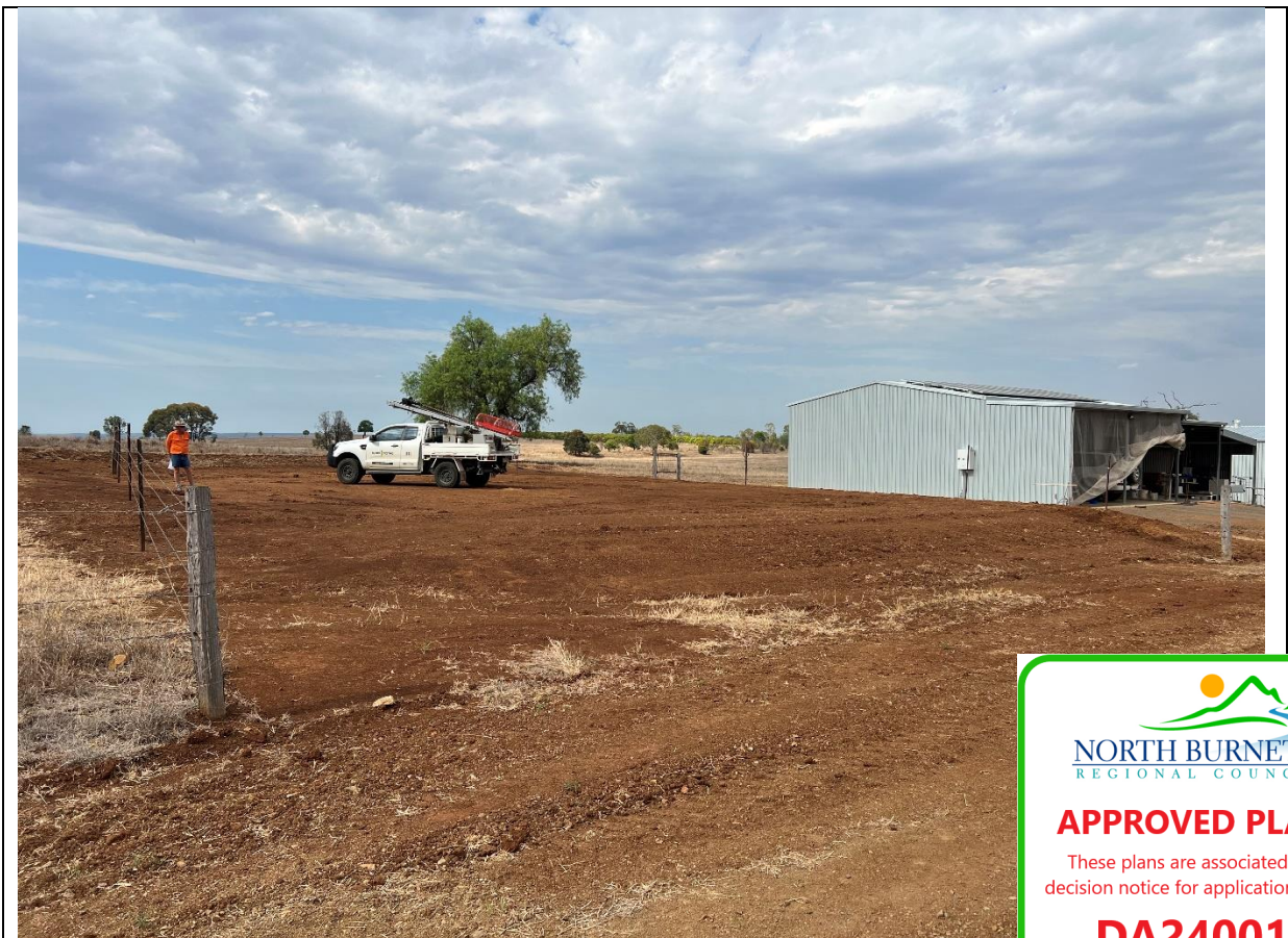
Image 2 – Proposed construction site
