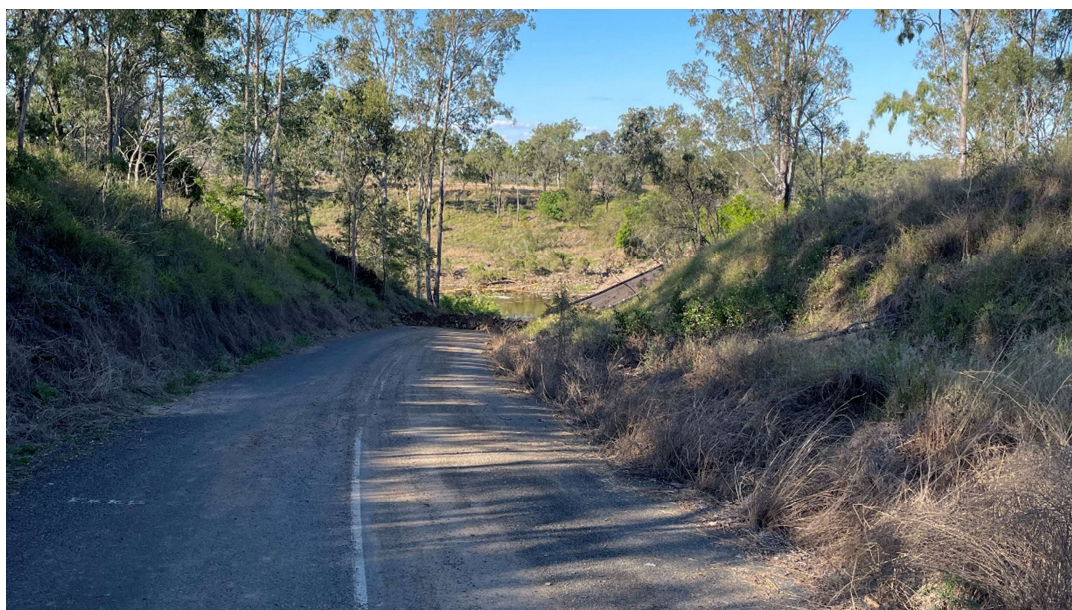
Figure 4: Western Approach to the Bon Accord Bridge (Give Way Side)
