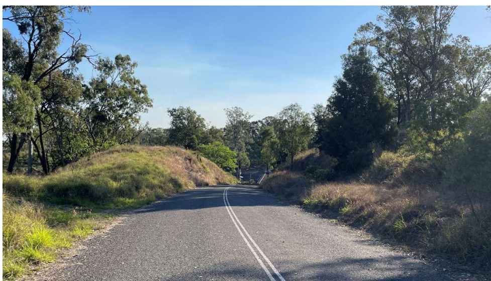
Figure 3: Eastern Approach to the Bon Accord Bridge (Continuous Side)
