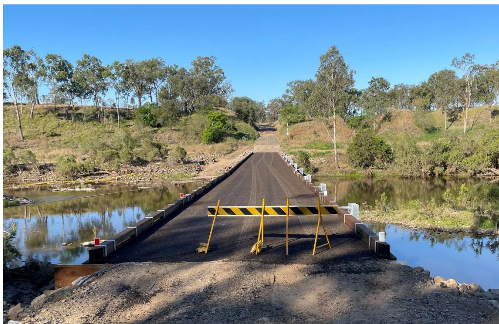
Figure 6: Existing Bridge No Linemarking
